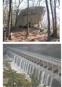
Photos of Indian Rock and the Gainer Dam Spillway courtesy of ProvWater.com
